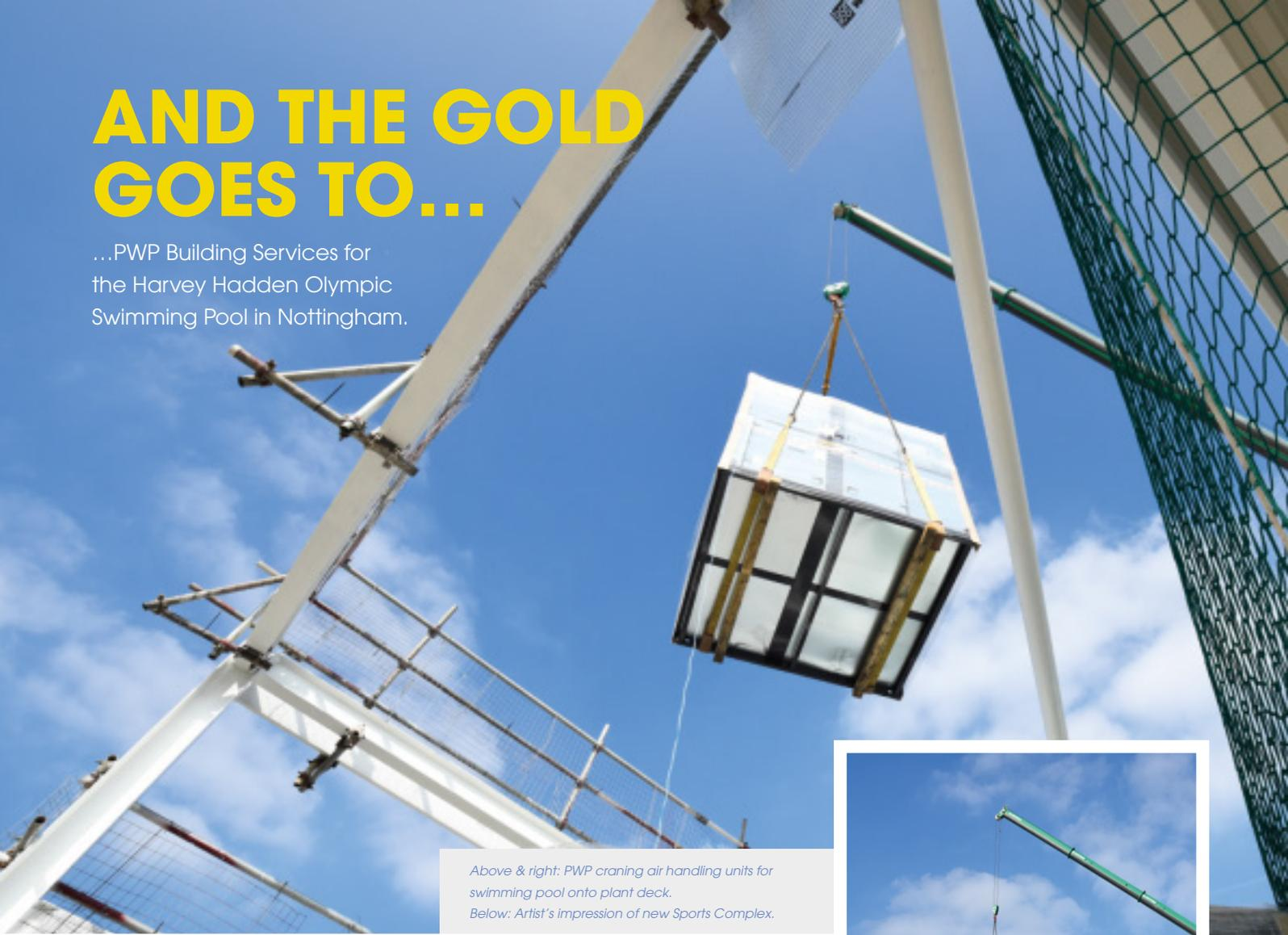
Above & right: PWP craning air handling units for swimming pool onto plant deck.
